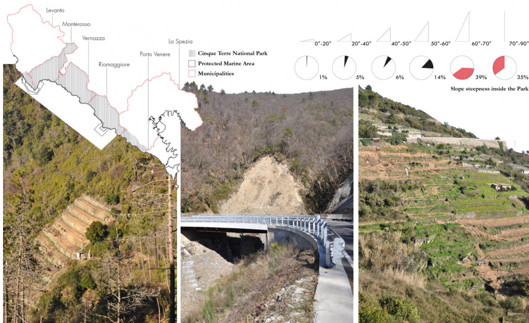
FIG. 1 The Cinque Terre National Park area and its steepness maintenance on new terraces in the national park area; a minor landslide over the SP370 road; renovation works on collapsed terraces after a heavy rainstorm above the village of Monterosso.
