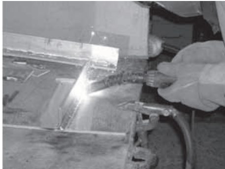
a) MIG “T” joint welding.
