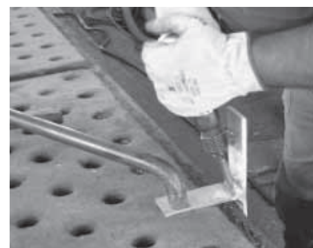
b) Hammer-peening of “T” joints.
