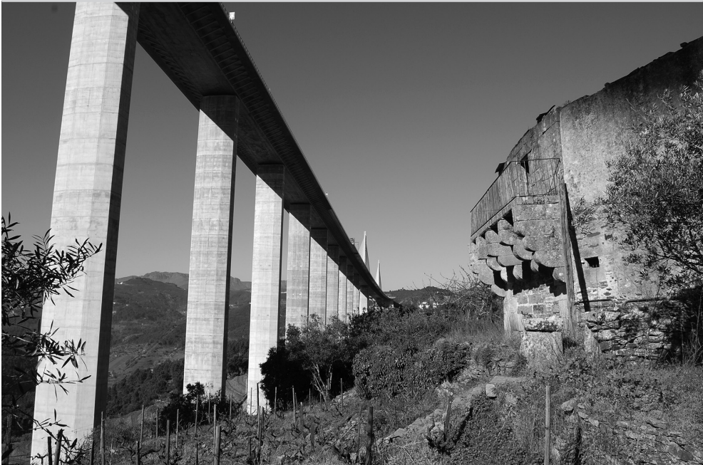
Figure 3 – The A24 highway bridge. Photo: Lorenzo Bordonaro.
