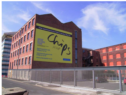
Figura 4 - Renovated industrial buildings - Ancoats, Manchester 2005 Steven Sarson
